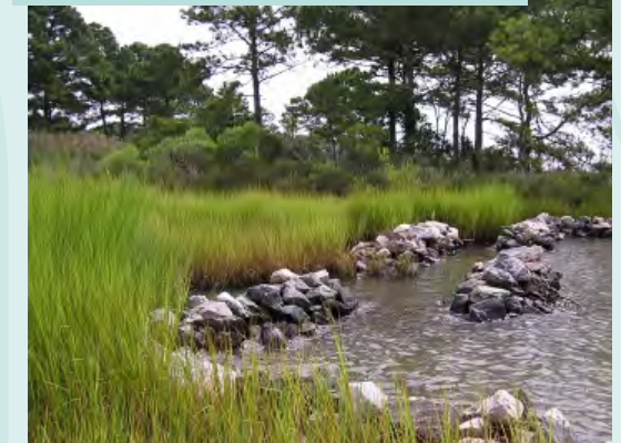
Source: Northeast Brandywine River Living Shoreline Project, Pennoni
