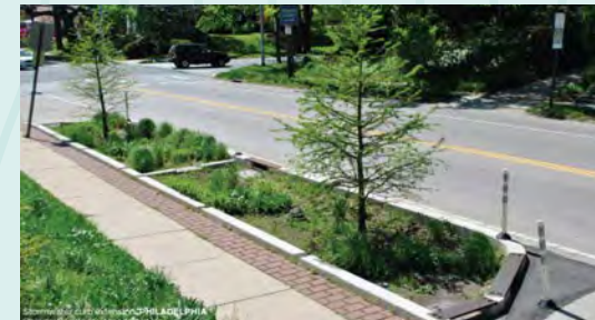
Stormwater tree trenches
